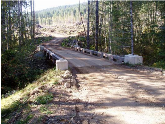
Permanent bridge and streamside tree retention, Tsable River area.
