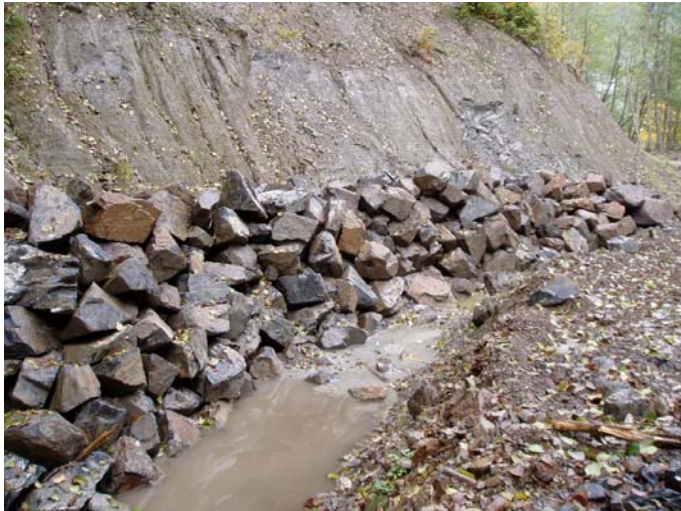
Rock used to stabilize cutbank at newly constructed road.
