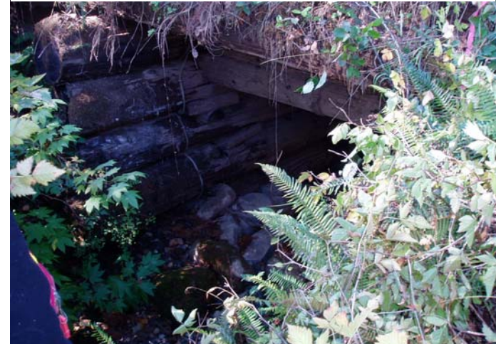
Structurally sound old wooden culvert.
