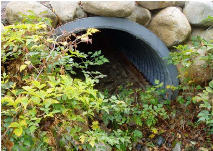
Open bottomed plate arch culvert.
