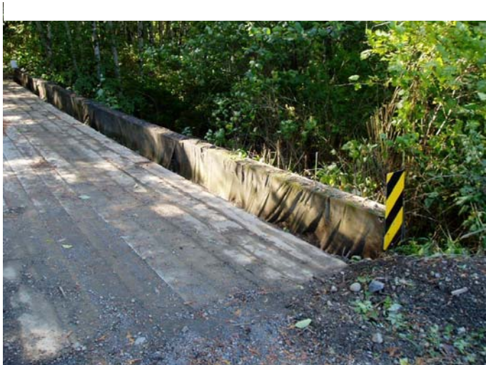
Filter cloth reduces sediment entering stream at bridge.
