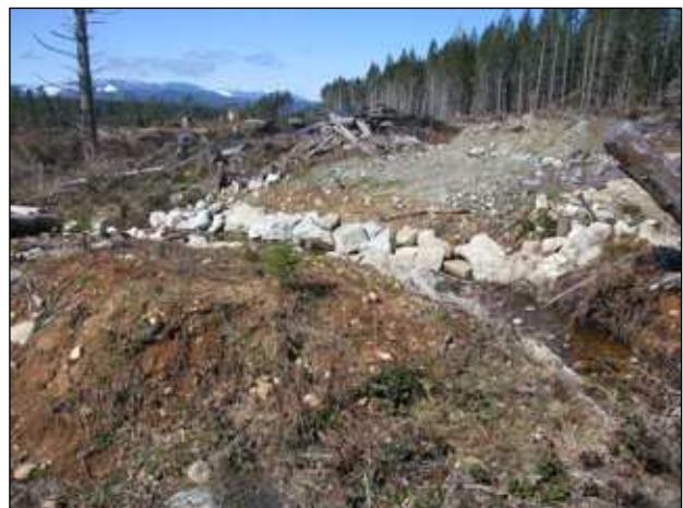
17. Culvert removed on deactivated road. Rip-rap remains in place to protect soil from erosion.
