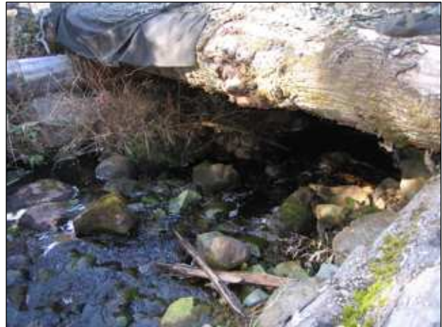
14. Wood culvert with sill logs well back leaving channel undisturbed. Note use of geo-fabric used to contain fines.
