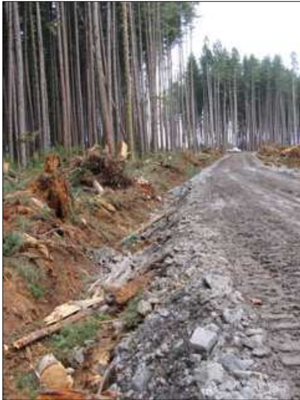
13. New road, ditch cleared of debris after right-of-way logs loaded out.
