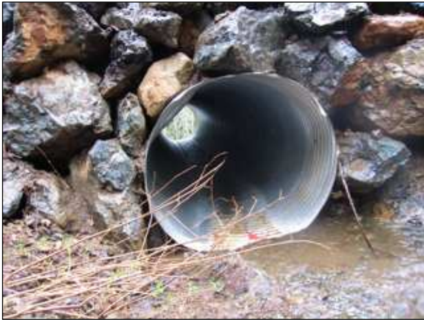
1. Culvert inlet armoured with placed shot rock.
