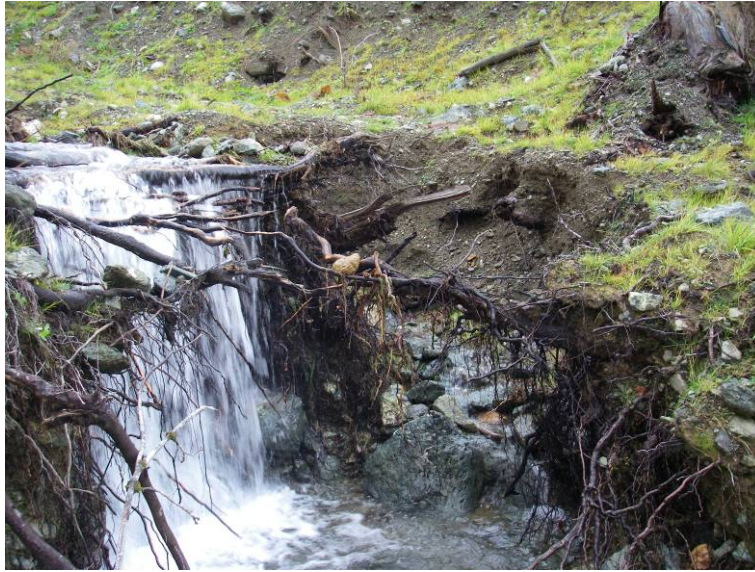
FIGURE 5. LOOKING UPSTREAM FROM C20 CROSSING (STREAM 6). TIMBERWEST HAS CLEARED THIS AREA OF SANDS, GRAVELS AND WOODY MATERIAL DEPOSITED IN THE NOVEMBER 2006 FLOOD. THE CHANNEL IS RE-GRADING TO A NEW, LOWER BASE LEVEL (SMALL 'KNICKPOINT' AT LOWER LEFT). THIS WILL CONTRIBUTE TO GENERATE SOME ADDITIONAL SEDIMENT UNTIL IT STABILIZES.
