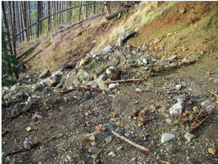
FIGURE 1. SHEET EROSION ON FORD BASE AT CROSSING C1 (STREAM 4). THE SURFACE IS NOW 'ARMORED' AS MOST ERODIBLE SOIL HAS BEEN REMOVED.
