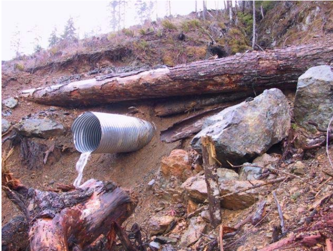
Outlet of culvert C1 (upper culvert) on stream 4.
