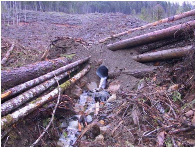
Outlet of culvert C11 (lower culvert) on stream 4.
