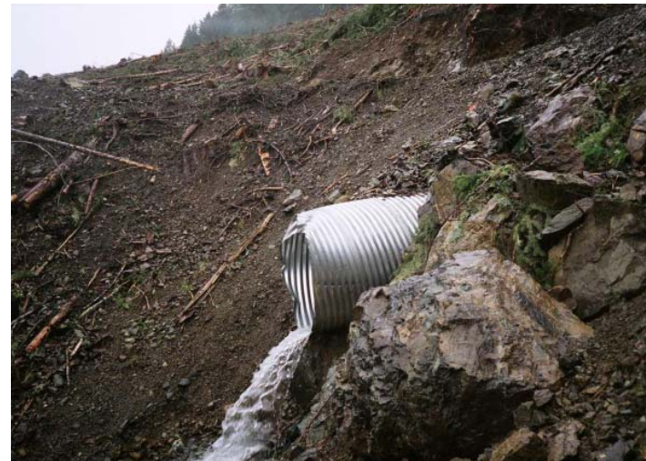
Outlet of culvert C27 on stream 6.
