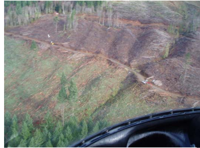
Overview of south west corner of block showing stream 4 and the replaced crossing C-11.
