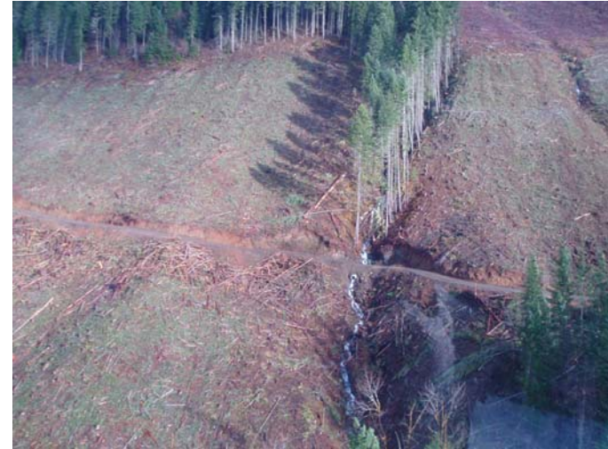
Crossing C-27 on stream 6 with stream reserve above.
