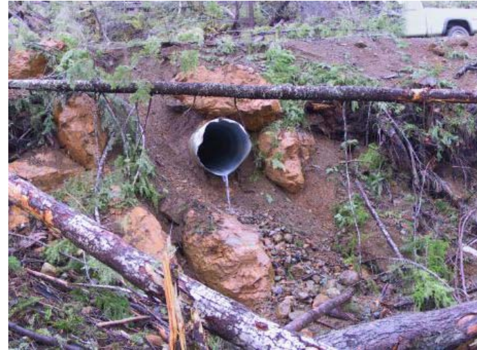
Outlet of culvert C18 (middle culvert) on stream 4.
