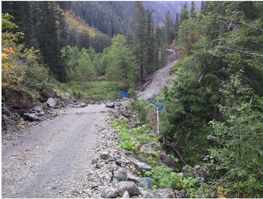
Photo 5 Looking at the upper road crossing of Kweishun Creek ( channel location marked with blue arrows).
