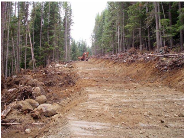
Excavator building a new road near Nelson
