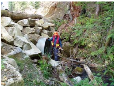
Shawn Hamilton inspecting a corrugated metal stream culvert at coastal site
